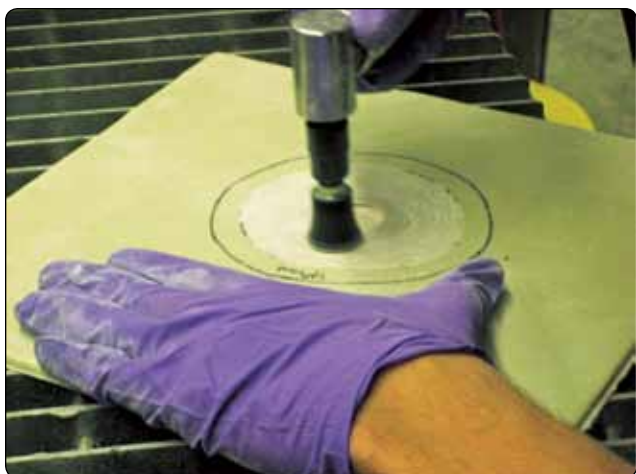
Figure 7-58. Taper sanding of repair area.
