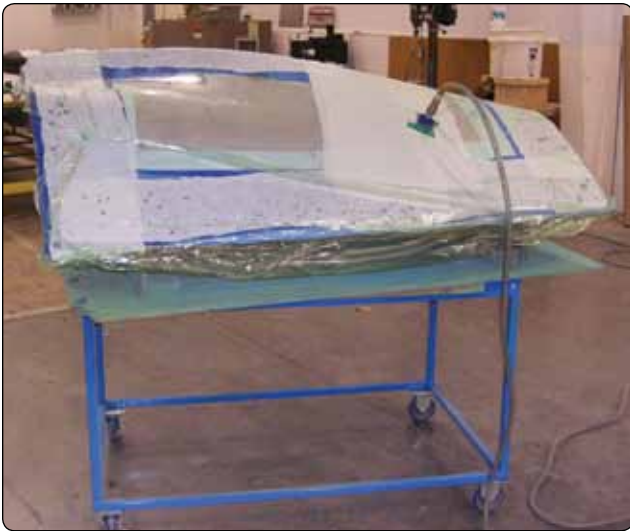
Figure 7-52. Envelope bagging of repair.
